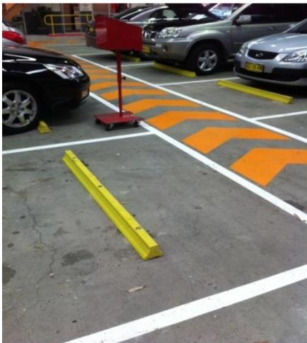
**Examples of alternative barriers to control vehicle and pedestrian access**
